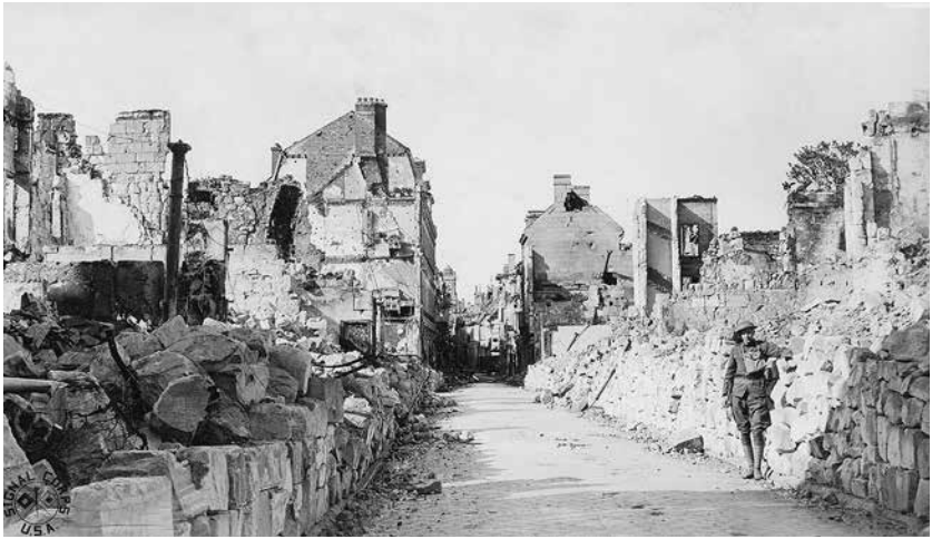
Street in Soissons, September 1918 (National Archives)
